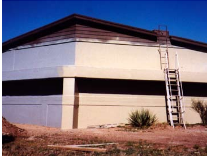
After: Repaired damage to concrete water reservoir. --- Mesa Verde National Park
