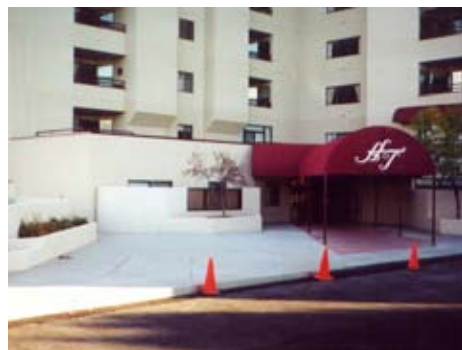
After: Repaired deck at Horizon Towers.--- Grand Junction, CO
