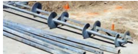
Helical piers ready for installation.
