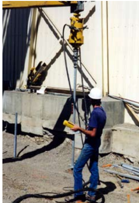
Helical piers for new industrial park.
