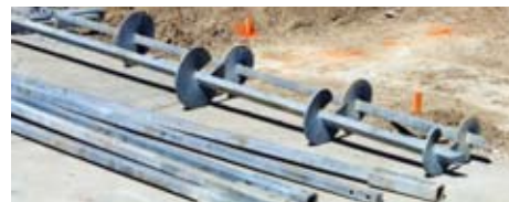
Helical piers ready for installation.
