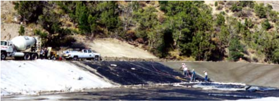
Shotcrete (approx. 400 cu. yards) utilized on retention pond for South Canyon Landfill. --- Glenwood Springs, CO
