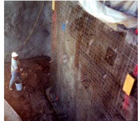
Permanent shotcrete wall (soil nailed wall) for basement addition. --- Aspen, CO
