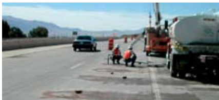
Slab-jacking used to raise and stabilize sections of I-70. -- CO
