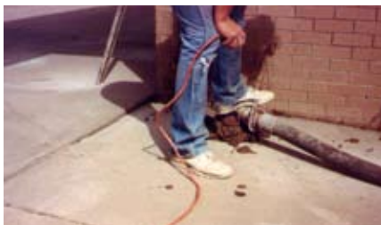
Quickly raising concrete slabs by pumping pressure injected grout beneath slab.
